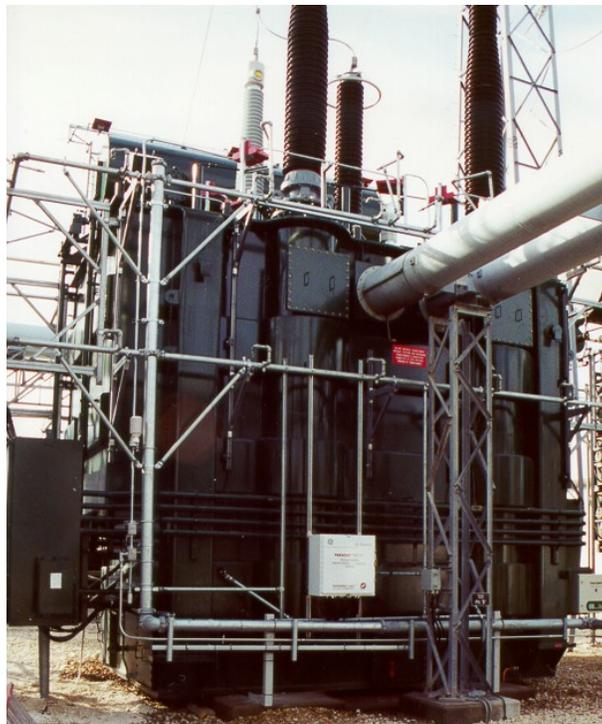
Figure 8 – Fiber optic temperature sensor on a 107MVA converter transformer
